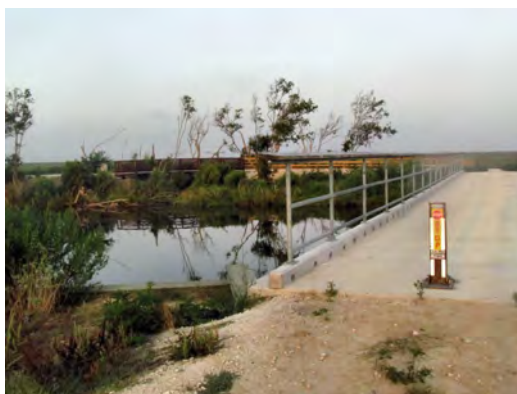
Cross the bridge and follow the sidewalk
